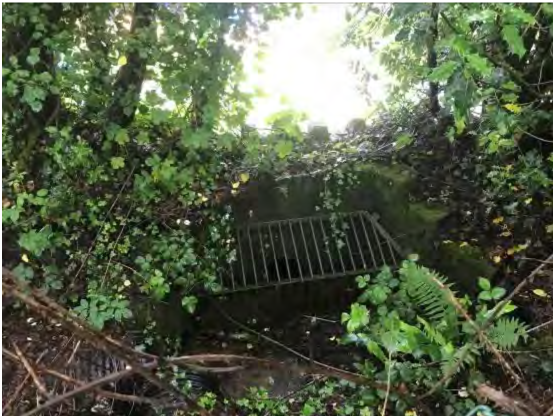
Photograph 36 – Inlet chamber at rear of school
