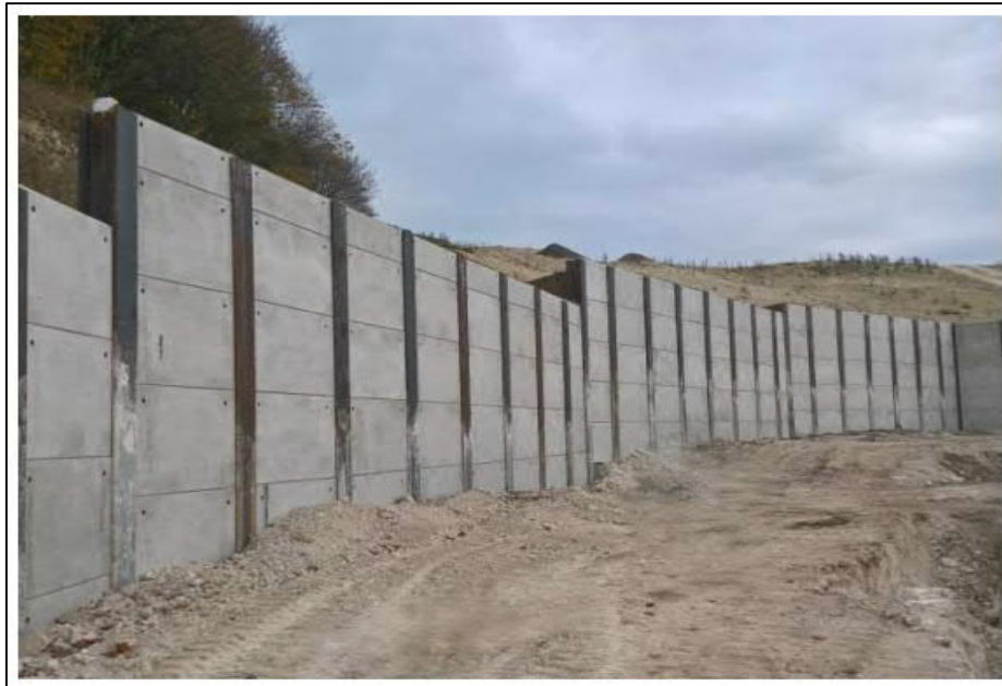
Insert 3: King Post Retaining wall example
