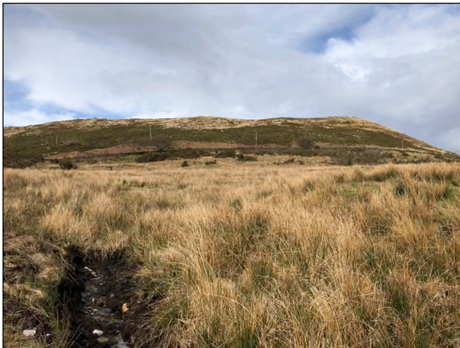
Plate 16: General view of landslide looking north.
