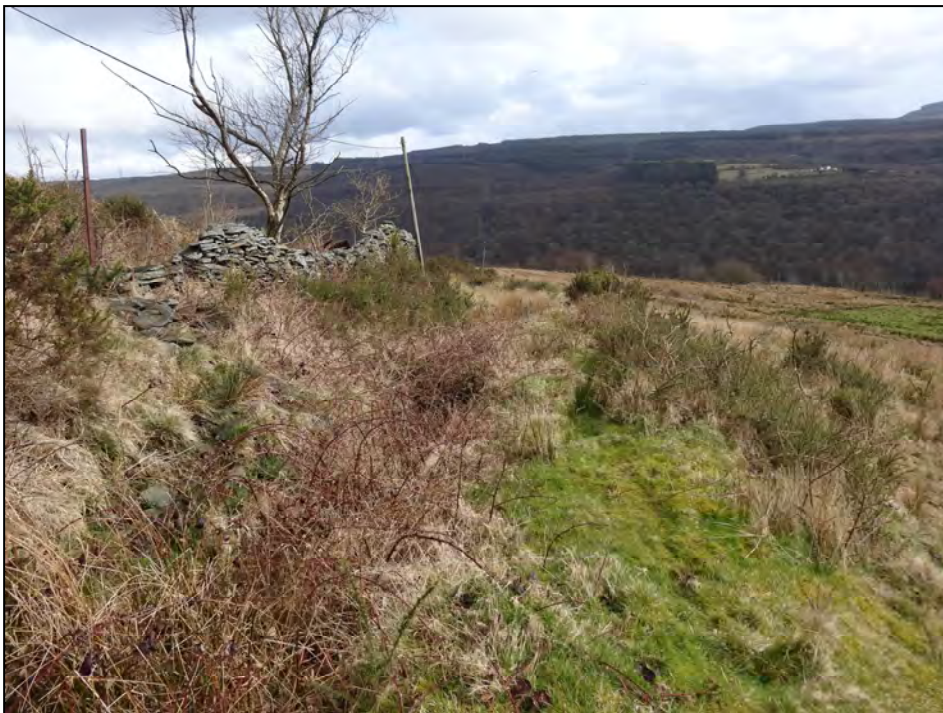
Plate 8: View along rear of landslide looking east. Note disturbed telegraph pole in middle distance and ditch in foreground.
