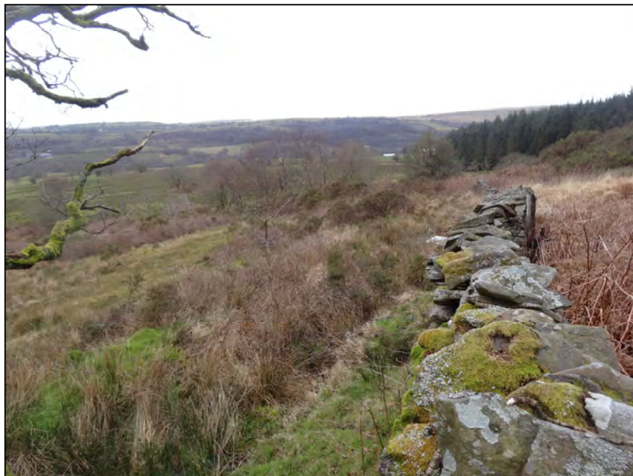
Plate 2: General view western area of the landslide, looking west along dry stone wall.
