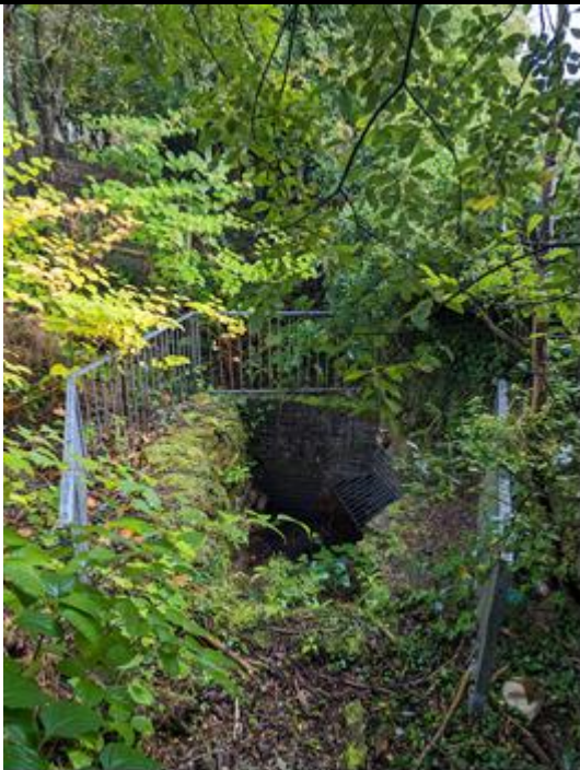
Plate 6: Feature S3 at ch. 0 – culverted watercourse.
