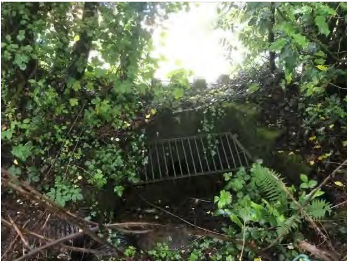
Photograph 36 – Inlet chamber at rear of school
