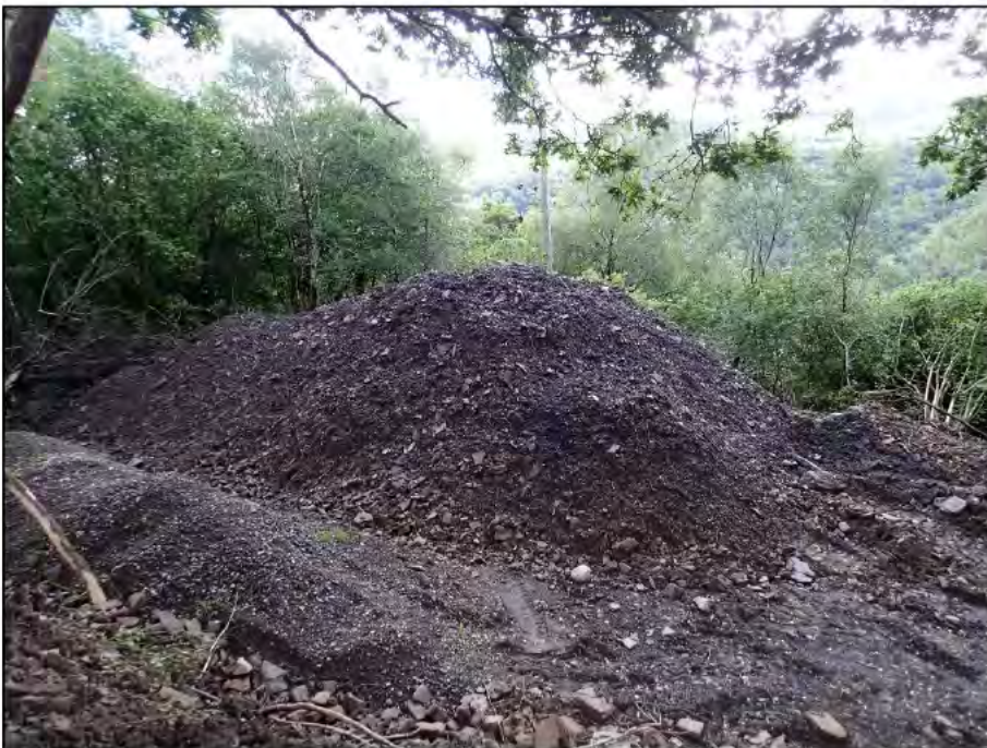
Plate 6: Recently deposited spoil from work in the quarry to the NW of the School.
