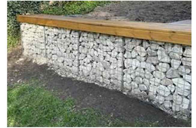
Image showing gabion basket retaining wall
