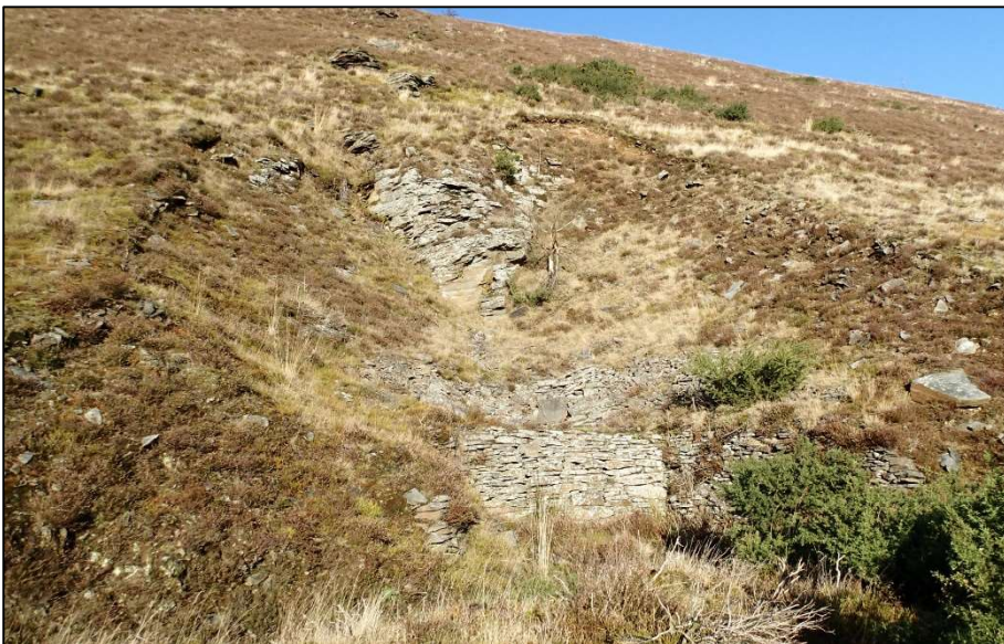
Plate 8: Shallow, small (<math><10\text{m}^3</math>) landslides above former adits in the No 2 Rhondda Seam.
