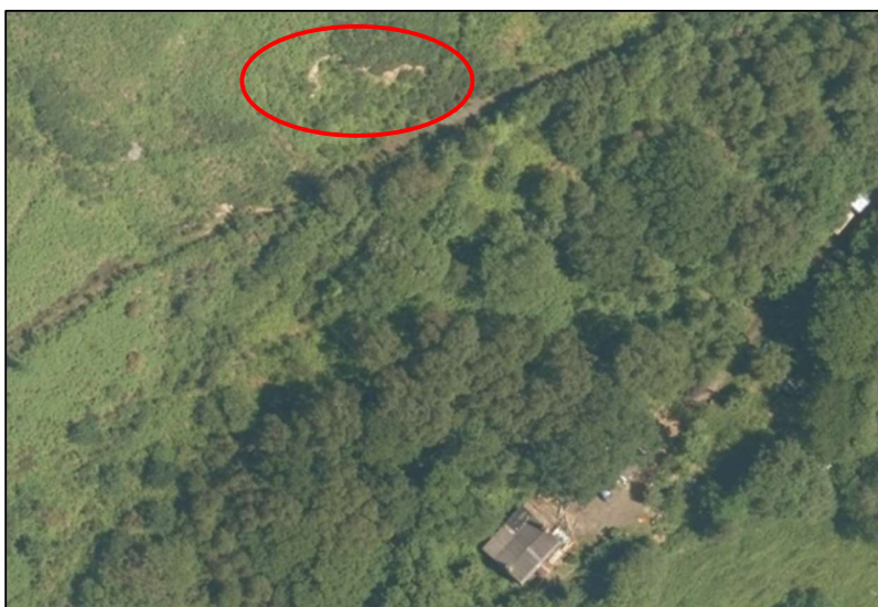
Figure 8: Tension crack (circled) above former adit location
