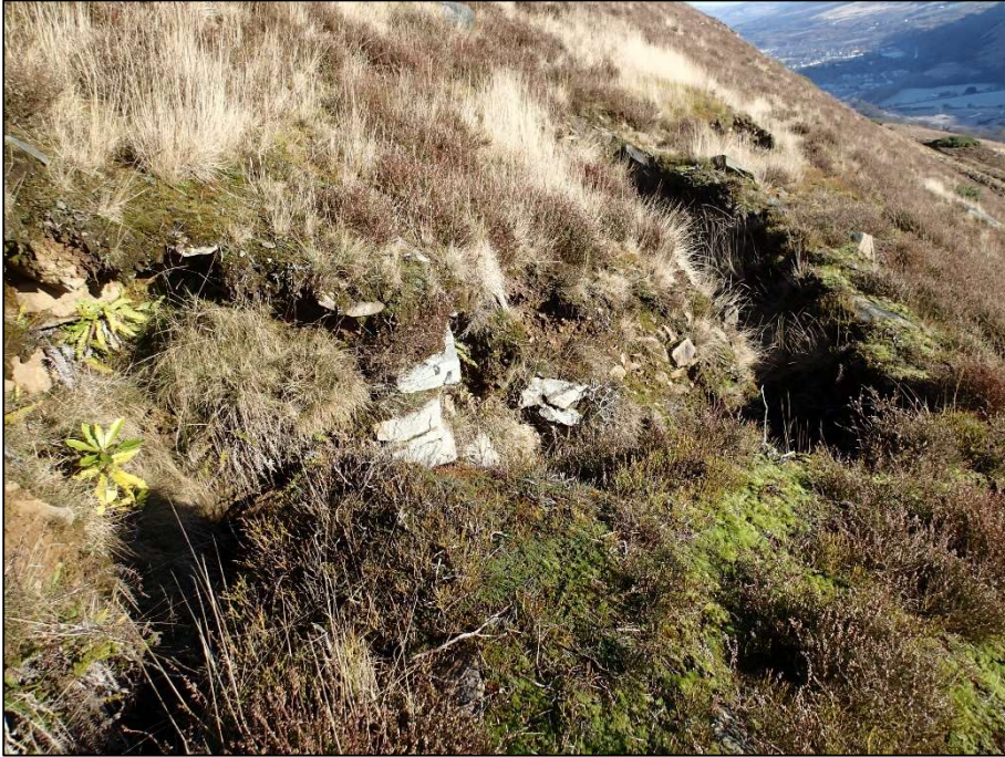
Plate 7: Tension crack above the No2 Rhondda coal seam likely to be the result of localised mining induced instability.
