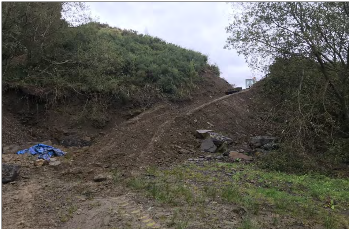
Plate 10: Overview of access track through former Cwar Pen-twyn Quarry (Q2), looking towards the west.
